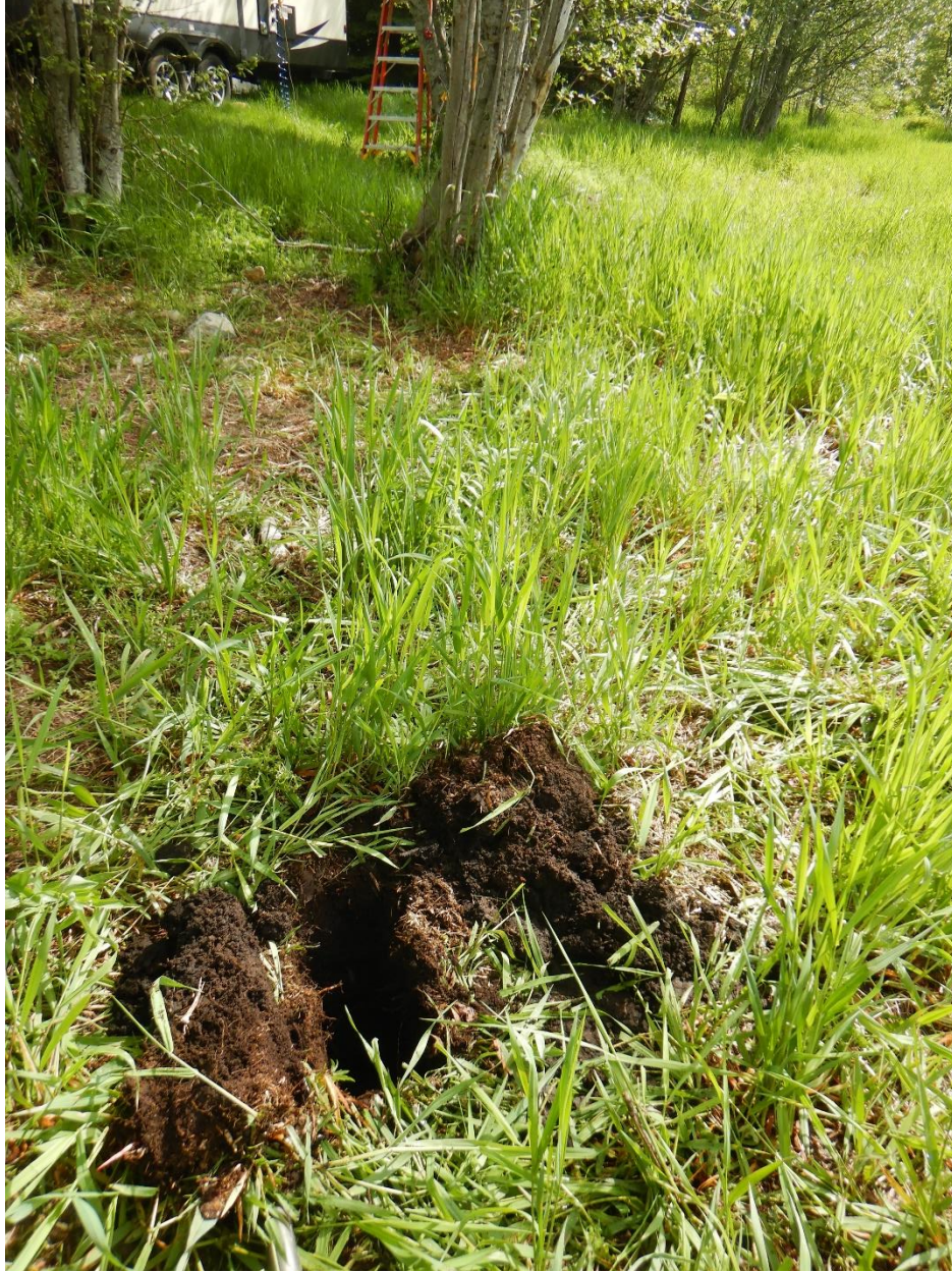
Photograph 4. SP1; wetland pit looking east.
